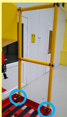
Figure 7: Railing installed on the step
